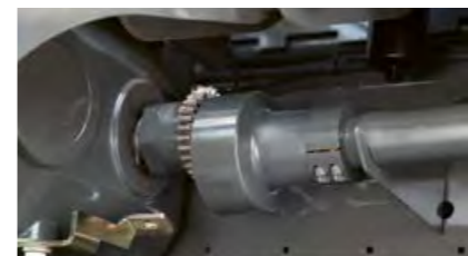
Disconnecting the drive shaft.
