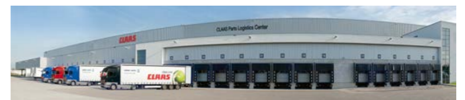
The CLAAS Parts Logistics Center in Hamm, Germany, stocks more than 155,000 different parts in a warehouse area of over 100,000 m 2 .
